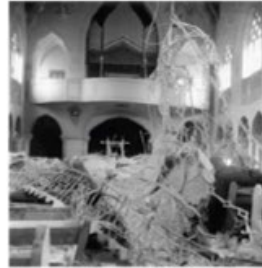
Figure 8: The 1946 earthquake of Sierrre: Photographs of the collapsed ceiling in the church of Chippis and of the landslide off the Rawylhorn, triggered by an aftershock of the earthquake, as well as a map of the inferred macroseismic intensities.
